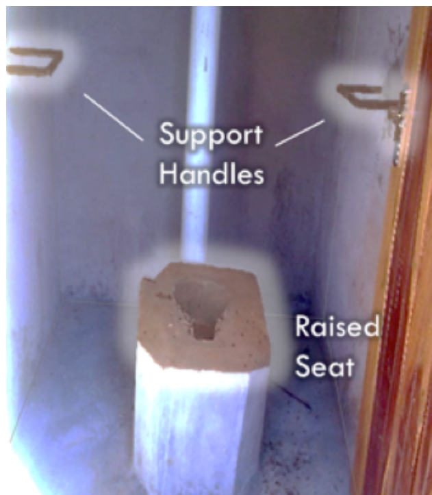
Disability friendly latrine at Makanda Primary School in Kasungu done by UNICEF implementing Partner 'Concern Universal' (photo credit, UNICEF Malawi)
