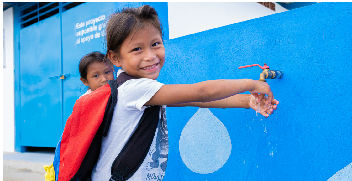
A girl washes her hands at the tap next to the Solar Water Treatment Plant installed by UNICEF in the community of San Francisco de Guayo, Delta Amacuro State, in the Bolivarian Republic of Venezuela.
