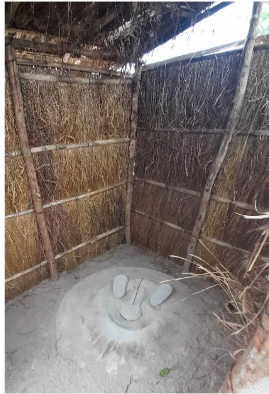
Figure 3.5: Cement slab to stand on in latrine, Metuge
