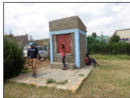
Picture 1: Water kiosk, Wukro
