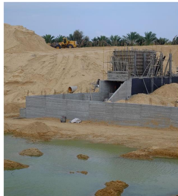
Construction of large infiltration pond in Gaza to support flood prevention
