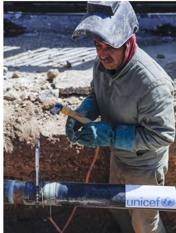
Rehabilitation of cisterns in the West Bank
