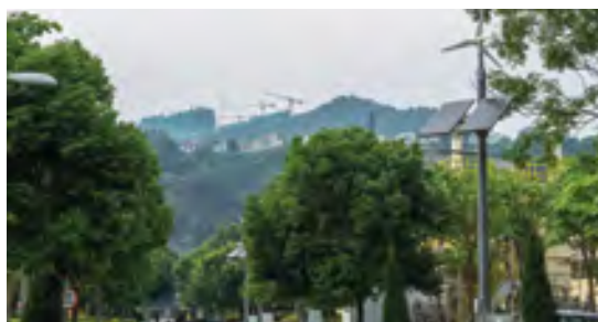
Solar panels and wind turbines power street lamps, Hong Kong, China
