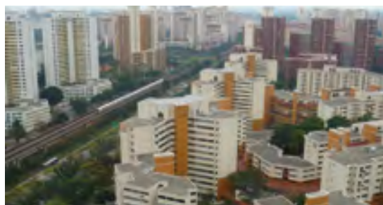
Affordable housing in Bukit Batok, Singapore
