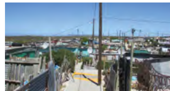
Street lights on the Monwabisi Park Informal settlement pedestrian walkway, Cape Town, South Africa
