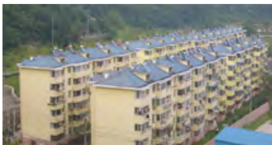
A new residential neighbourhood equipped with solar water heaters, Tieshan, Hubei, China
