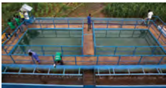
Employees work at the Bentiu water treatment plant, South Sudan
