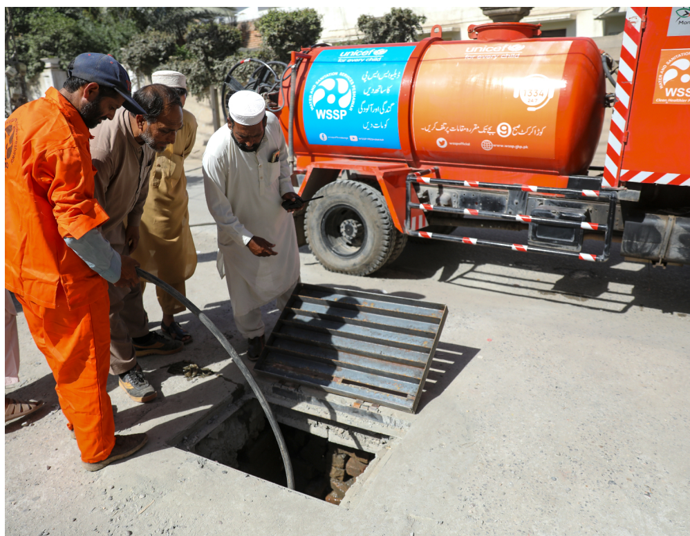
Water and Sanitation Services Peshawar workers open a sewer line with the help of a UNICEF-supported sewer rodding machine in Gulberg # 2, Peshawar, Khyber Pakhtunkhwa Province, Pakistan.
